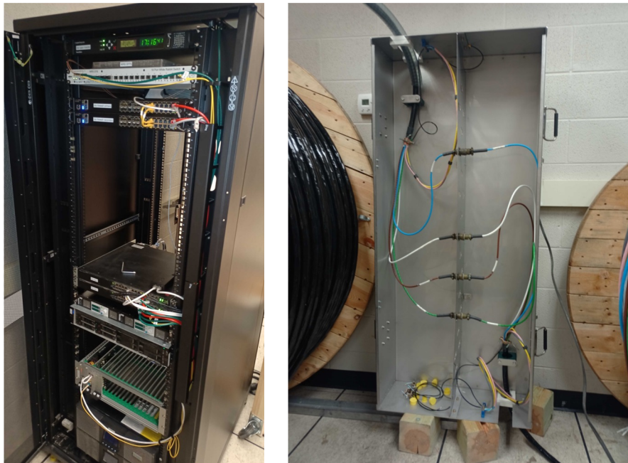
NTS - Upgrade cabling systems
